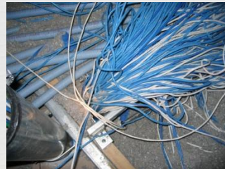
Example of existing wiring on 2 nd floor.
