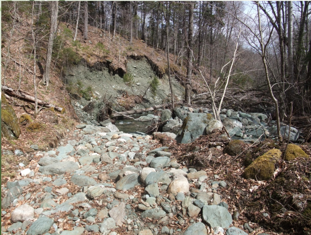
Tunnel Brook Before
