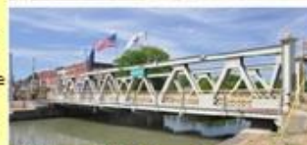
Middleport Lift Bridge, 1915 and Today.
